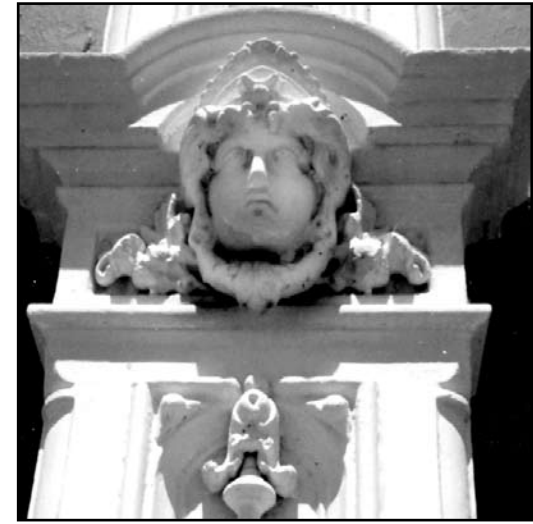
Above: A detail of the Cast Iron column on the Albany Regional Museum Building. The face is said to represent Minerva the goddess of wisdom, and was cast in Albany at the Albany Iron Works. The column has since been painted black.
