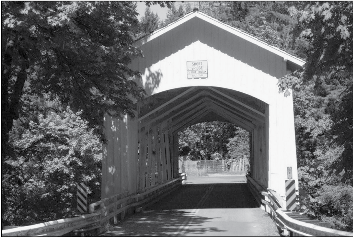
Short bridge over the South Santiam River. Photo by: Cathy Webb.
