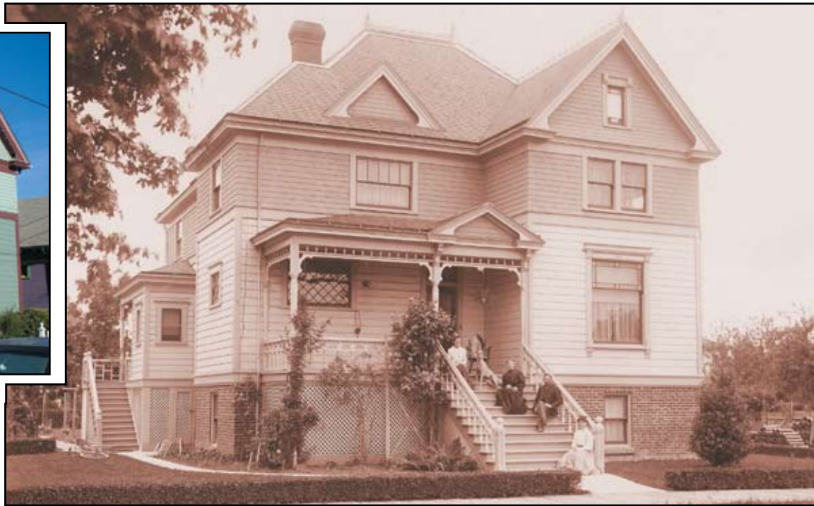
Above photo: Courtesy of Randy and Jody Kruse. The Buhl house (8) originally had a basement but was moved after 1912 to the current location at Seventh and Montgomery to a foundation without a basement. It may have been built as early as the 1880s. Photo c. 1911 Shows Mr. & Mrs. H.C. Harkness, their daughter Ora, who the house was named after, Ora's aunt and the family dog, a great dame. Ora lived in the house until she was 92.
